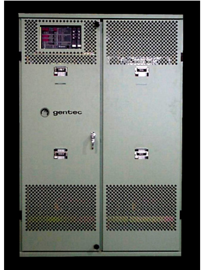
Redundant Battery Charger 125 VDC, 150 A
